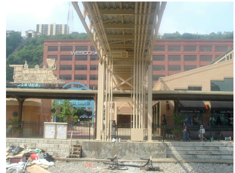
MEP System Under The Pedestrian Bridge
