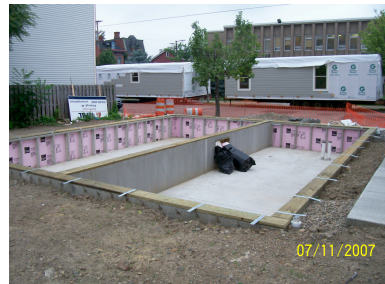
Foundation For a UFAS Compliant Two-Bedroom Modular Unit
