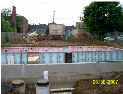
Foundation For A Three-Bedroom UFAS Compliant Modular Unit
