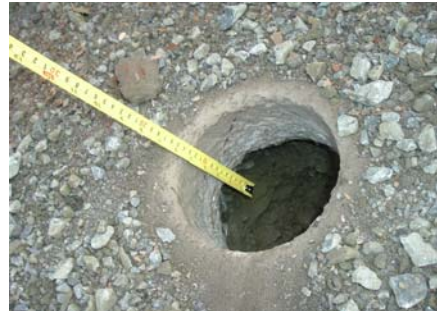
Landing Zone Pavement Cross-Section
